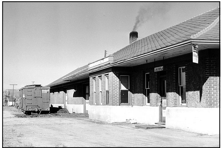
The railroad operation at Gunnison was extremely dead. After the station agent came to work, I found nothing would be running that day. Maybe the agent felt sorry for me, as he took me to the roundhouse. The yard was full of empty coal and stock cars. Bert Prall took this view in the Fall of 1953.
